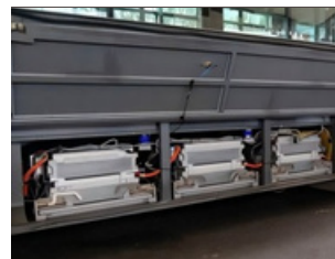
Public bus capacitor group/ lithium battery group
